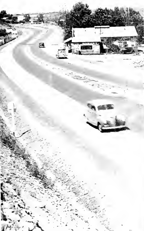
Views of channelization project recently completed on U. S. 99 near Redding that converted the existing 2-lane road into a 4-lane divided highway. At the 3-way intersection with Route 20 and the highway to Volcanic National Park, opposing traffic is separated by irregular shaped division strip areas partially bounded by concrete curbs.
